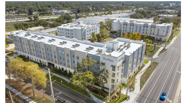
66 Units, $26.8M TDC
