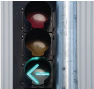
Modify existing traffic signal phasing to change from permitted to protected only phasing
