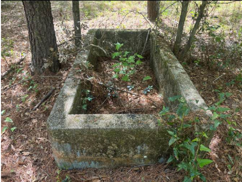
Photo 11 - Poured concrete cattle watering trough
