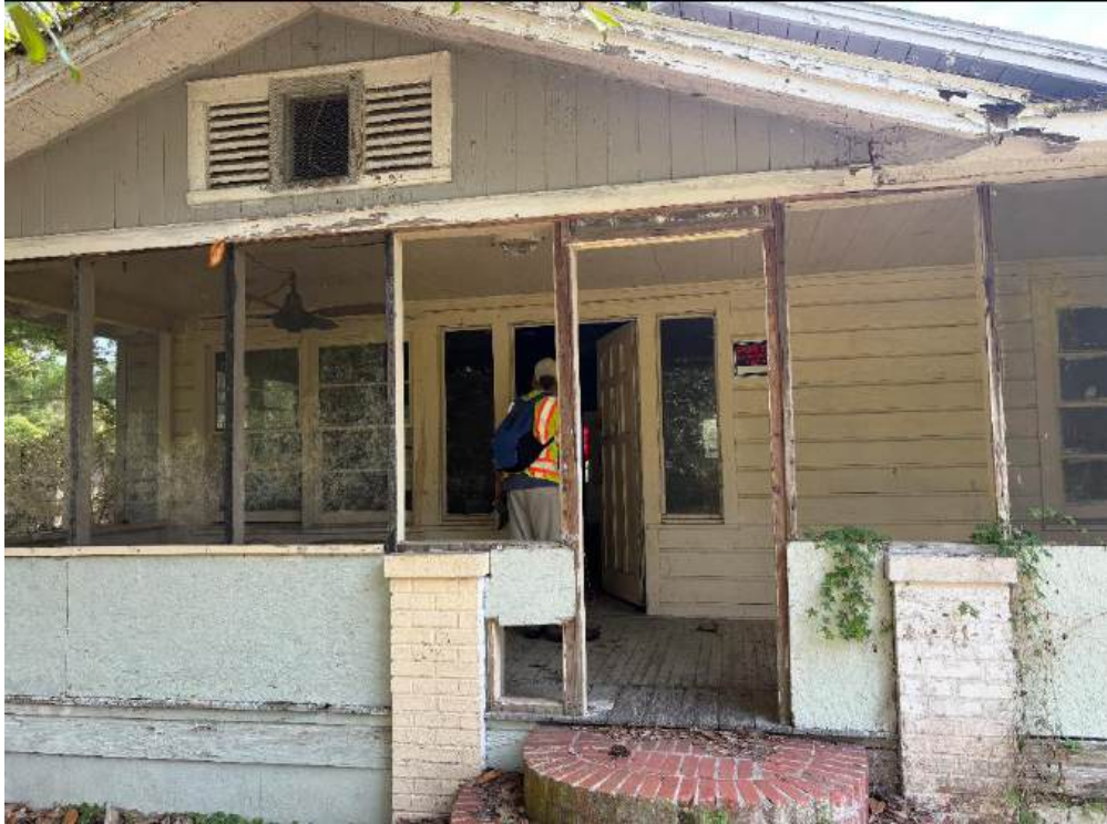
Photo 13 - Abandoned frame vernacular structure c. 1957 (8AL07618)
