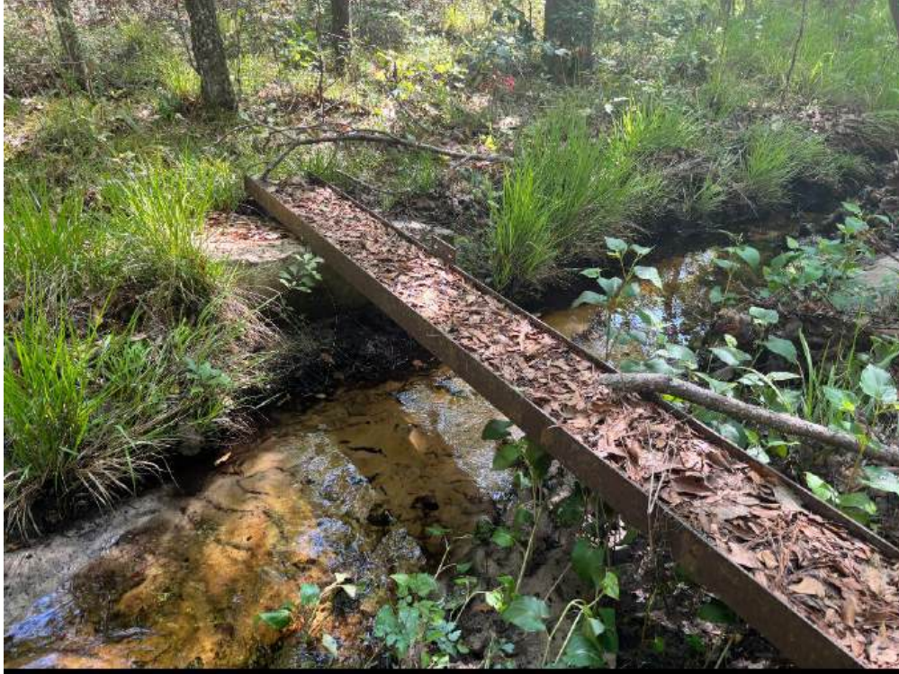
Photo 3 - Improvised metal beam bridge crossing over interior creek
