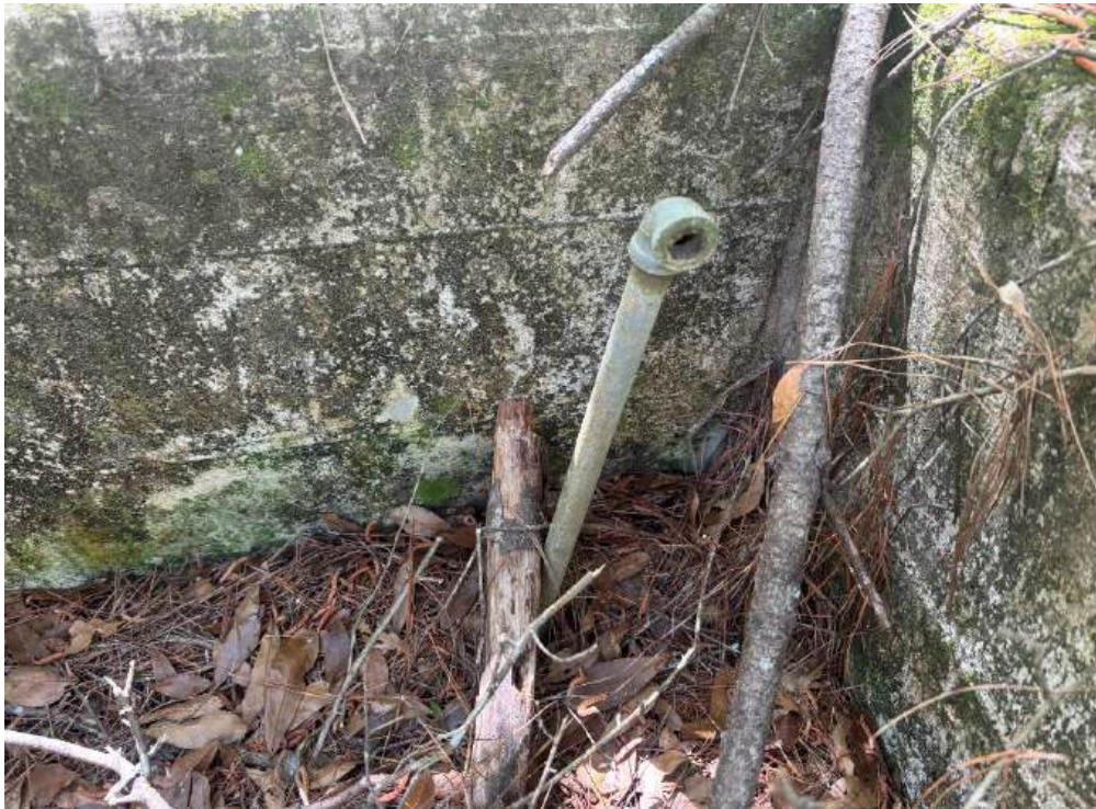
Photo 12 - Concrete cattle watering trough showing capped artesian wellhead
