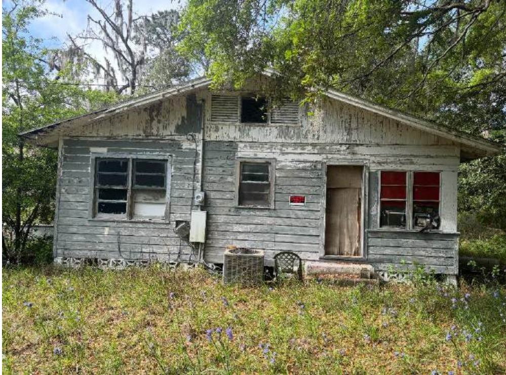
Photo 15 - c. 1957 historical structure in an advanced state of disrepair
