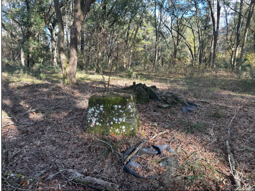
15 - Old Foundation Concrete Debris
