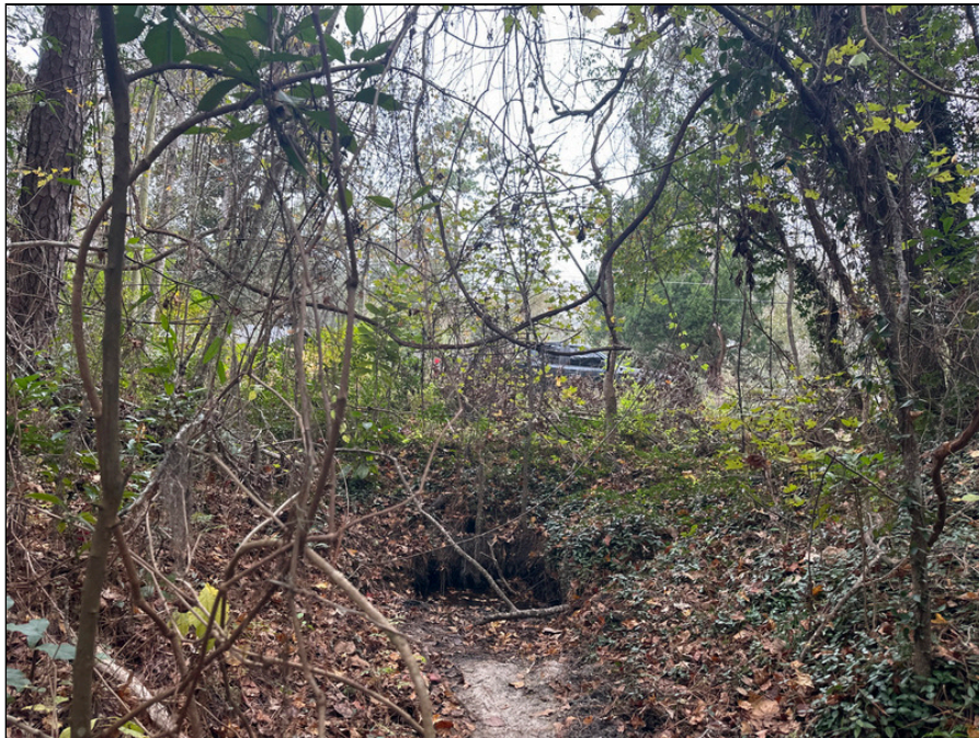
12 - Culvert along western border at 51st St OSW-A
