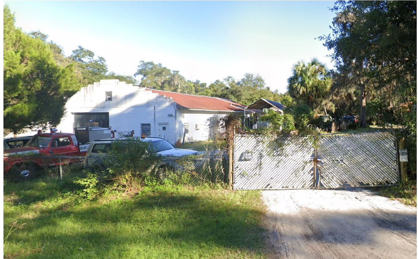
Existing commercial use frontage near SE Hawthorne Rd
