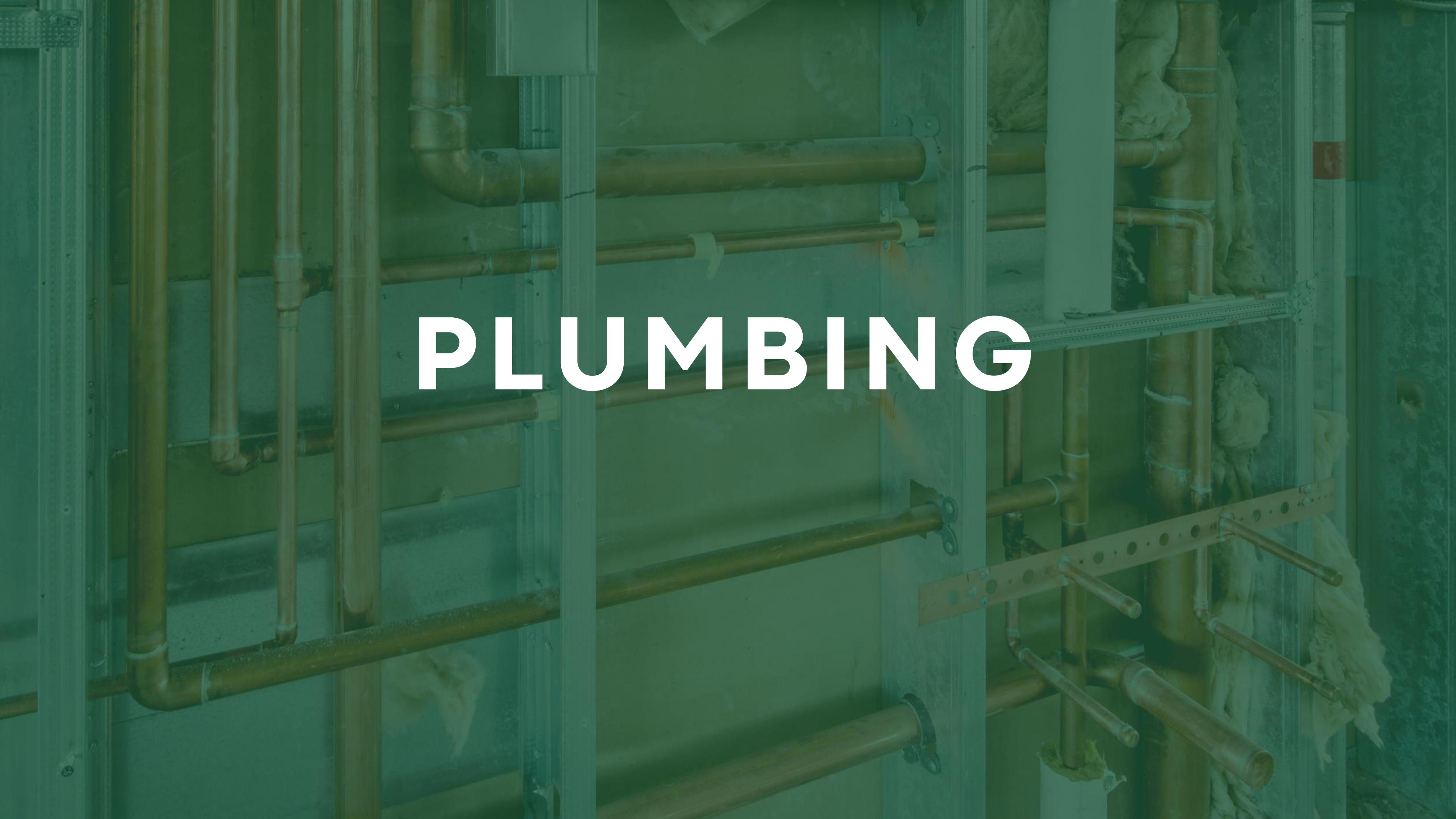
A photograph showing a dense network of copper pipes and insulation within a wall or ceiling structure. The pipes are primarily copper, with some white plastic components. They are secured to a light-colored wooden joist or wall studs with metal straps. The insulation consists of white mineral wool or fiberglass batts. The overall appearance is that of a professional plumbing or HVAC installation.
