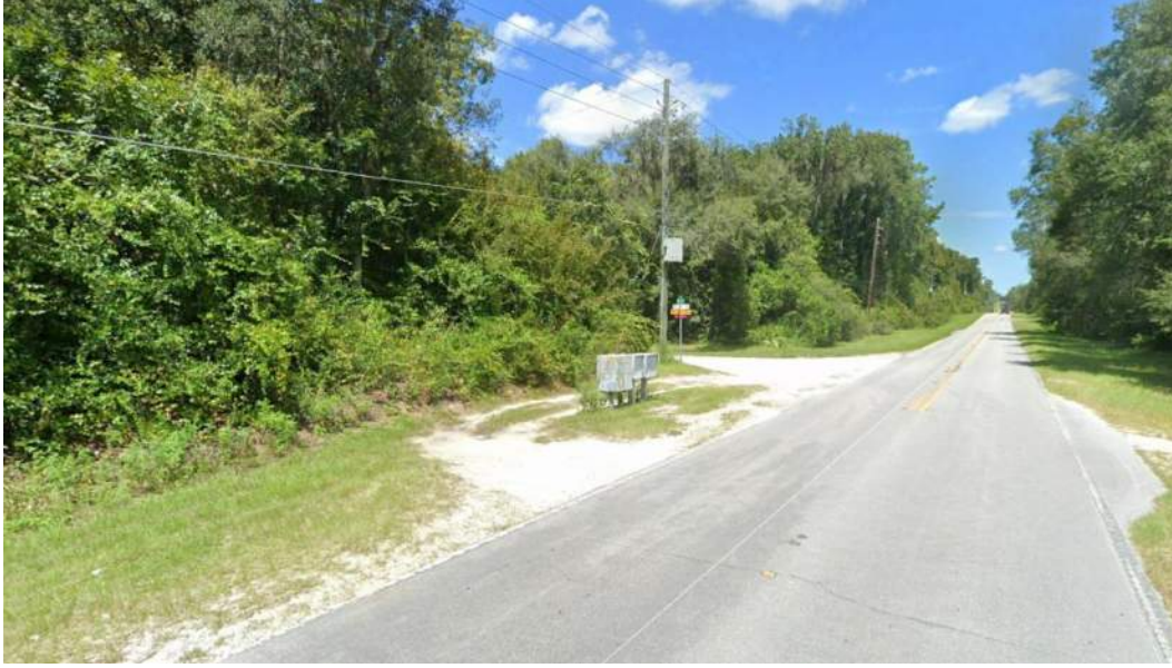
Figure 6-2 SE 30th Pl. Roadside Slope (Looking NW)
