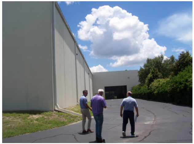
VIEW OF WAREHOUSE - NORTHEAST ELEVATION
