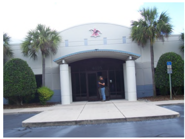
FRONT ENTRANCE TO OFFICE BUILDING
