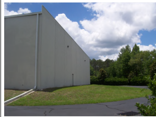
VIEW OF WAREHOUSE - NORTH ELEVATION
