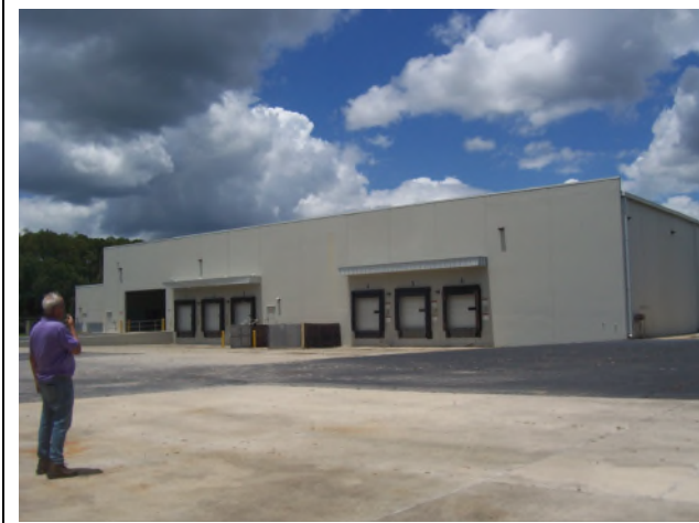
VIEW OF WAREHOUSE - SOUTH ELEVATION LOADING DOCK AREA
