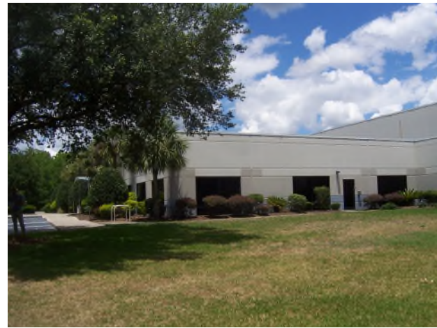
NORTHEAST VIEW OF OFFICE BUILDING
