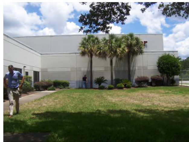
VIEW OF WAREHOUSE - SOUTHWEST ELEVATION
