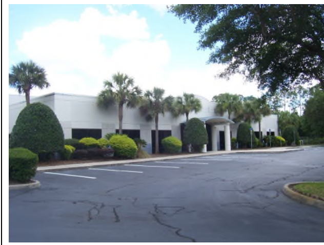
FRONT VIEW OF OFFICE BUILDING
