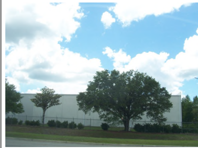
VIEW OF WAREHOUSE - WEST ELEVATION
