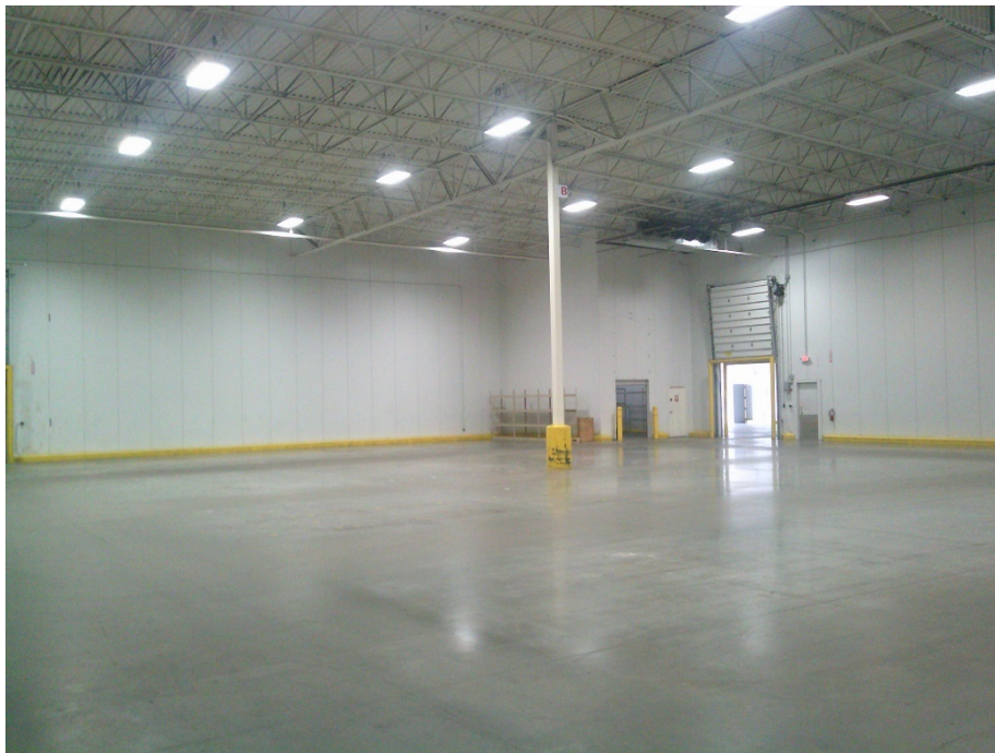
View of the air-conditioned warehouse area.
