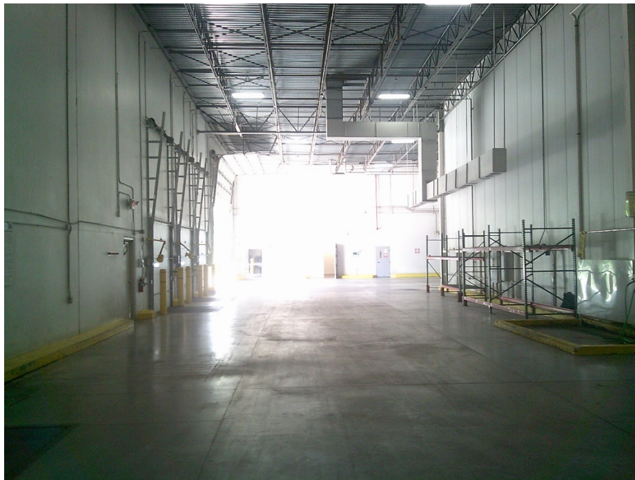
View of the loading dock area looking towards the office area.
