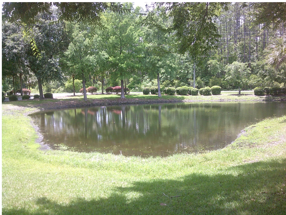
View of the retention pond located in the southeast corner of the property.
