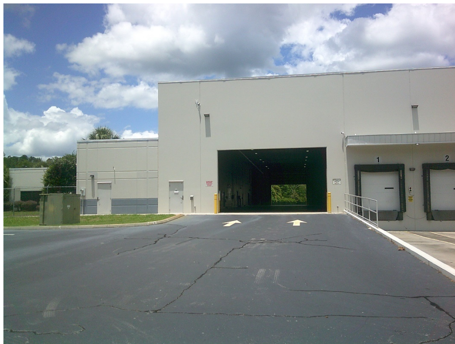
View of the rear of the building's drive-thru area.
