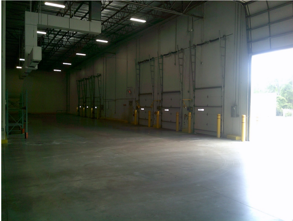
View of the loading dock area.
