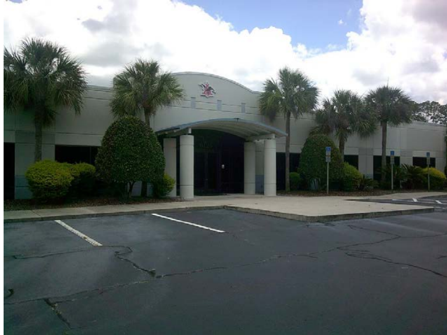
View of the front elevation of the office.
