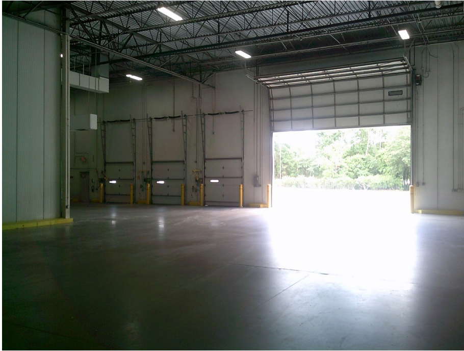
View of the warehouse area looking towards the loading docks.
