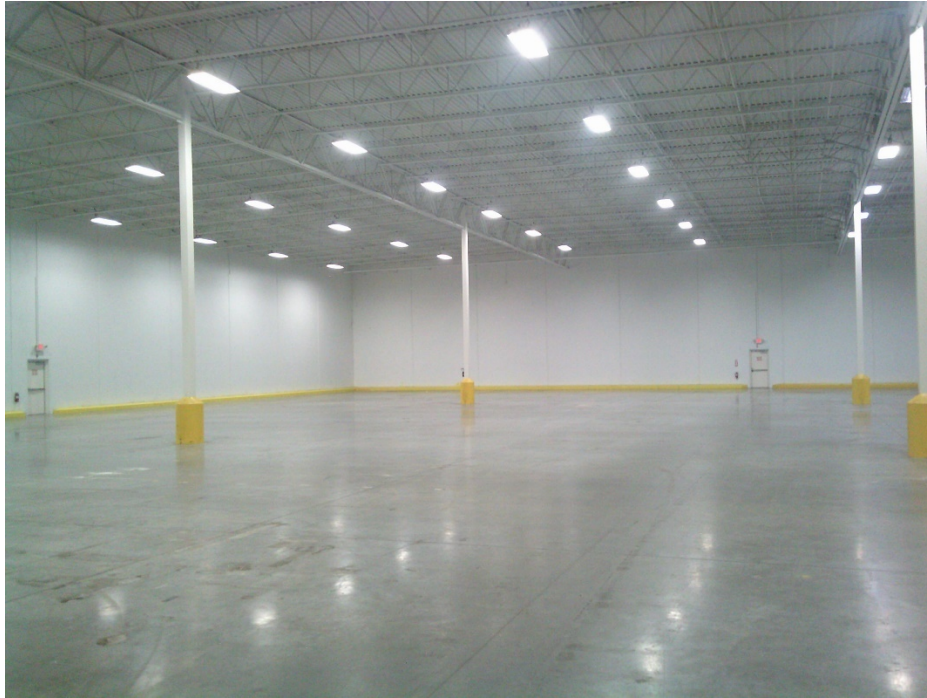
View of the air-conditioned warehouse addition area.
