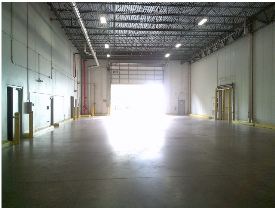
View of the warehouse area which is the former drive-thru.
