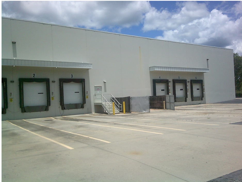
View of the rear of the building and the loading docks.
