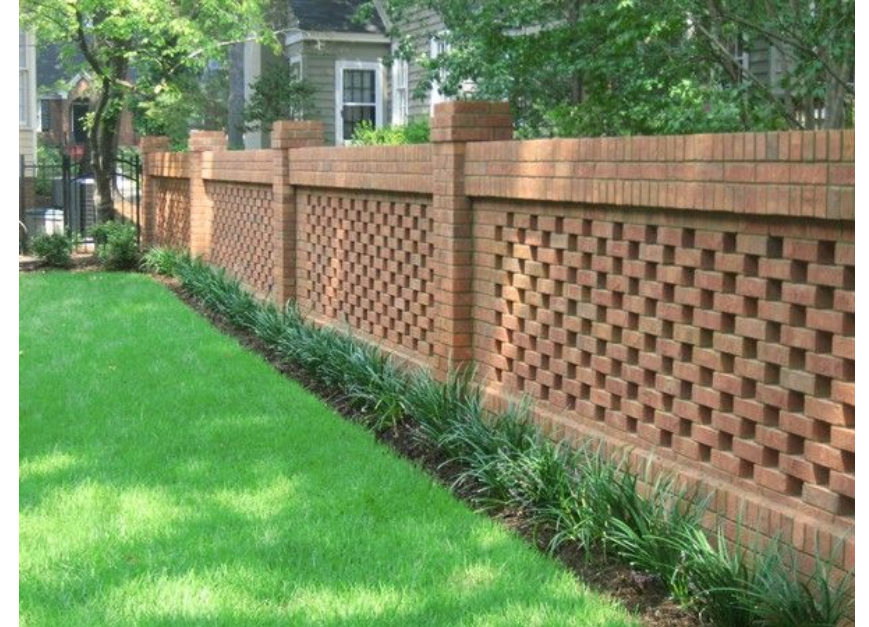
Multifamily property owners must construct and maintain a decorative masonry wall if their property abuts a single-family home.
