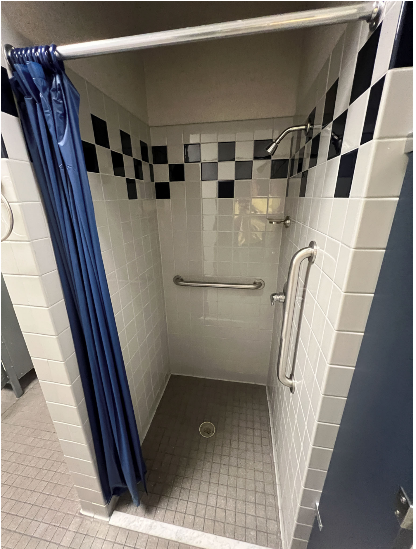
Shower needs hand held sprayer & fold down seat to make handicap
