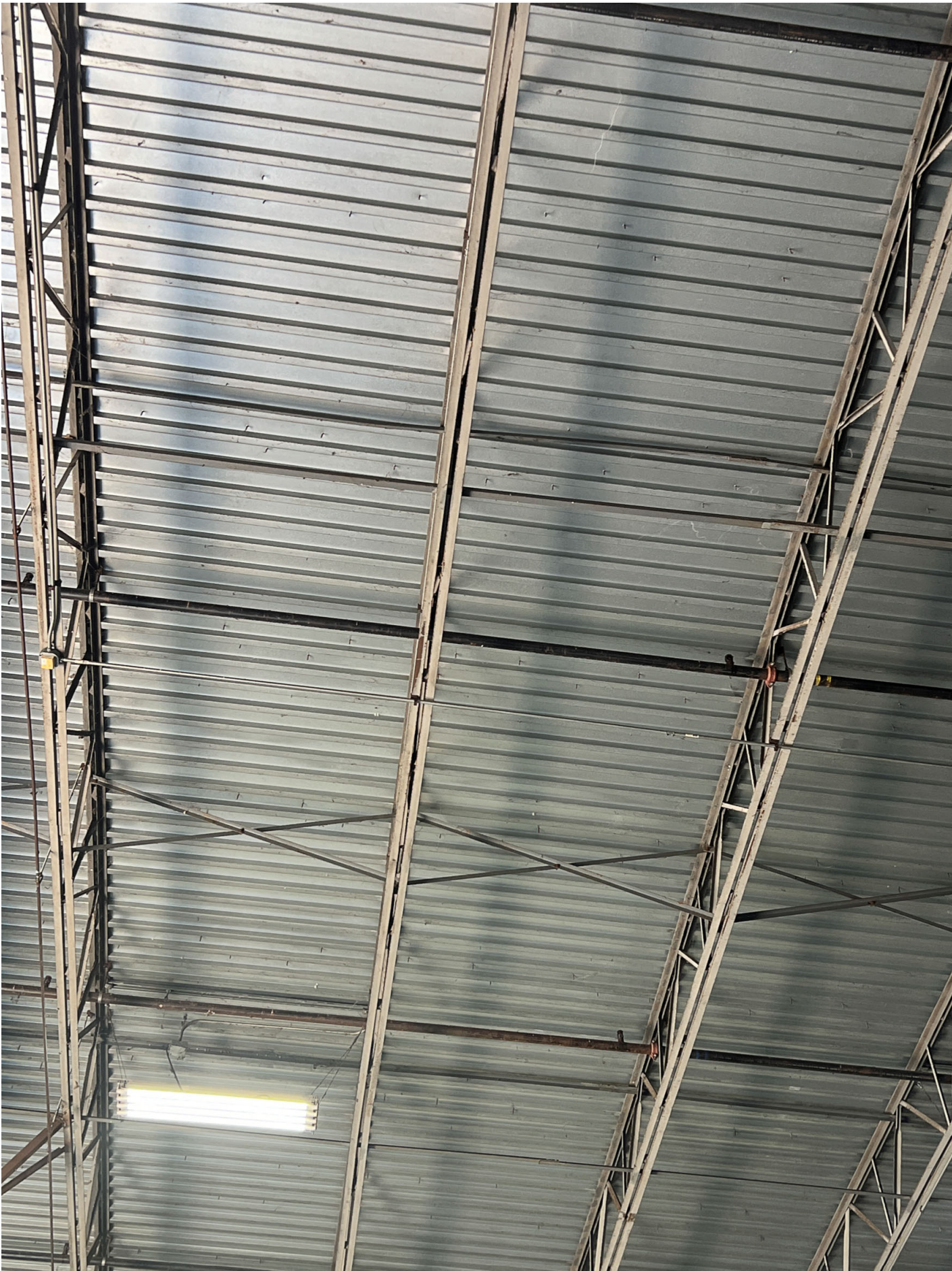
Joist with metal "B" deck roof structure
