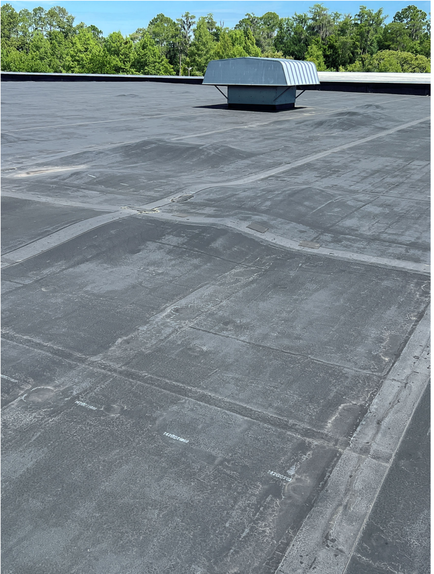
2000 warehouse roof large vapor bladder across the roof area
