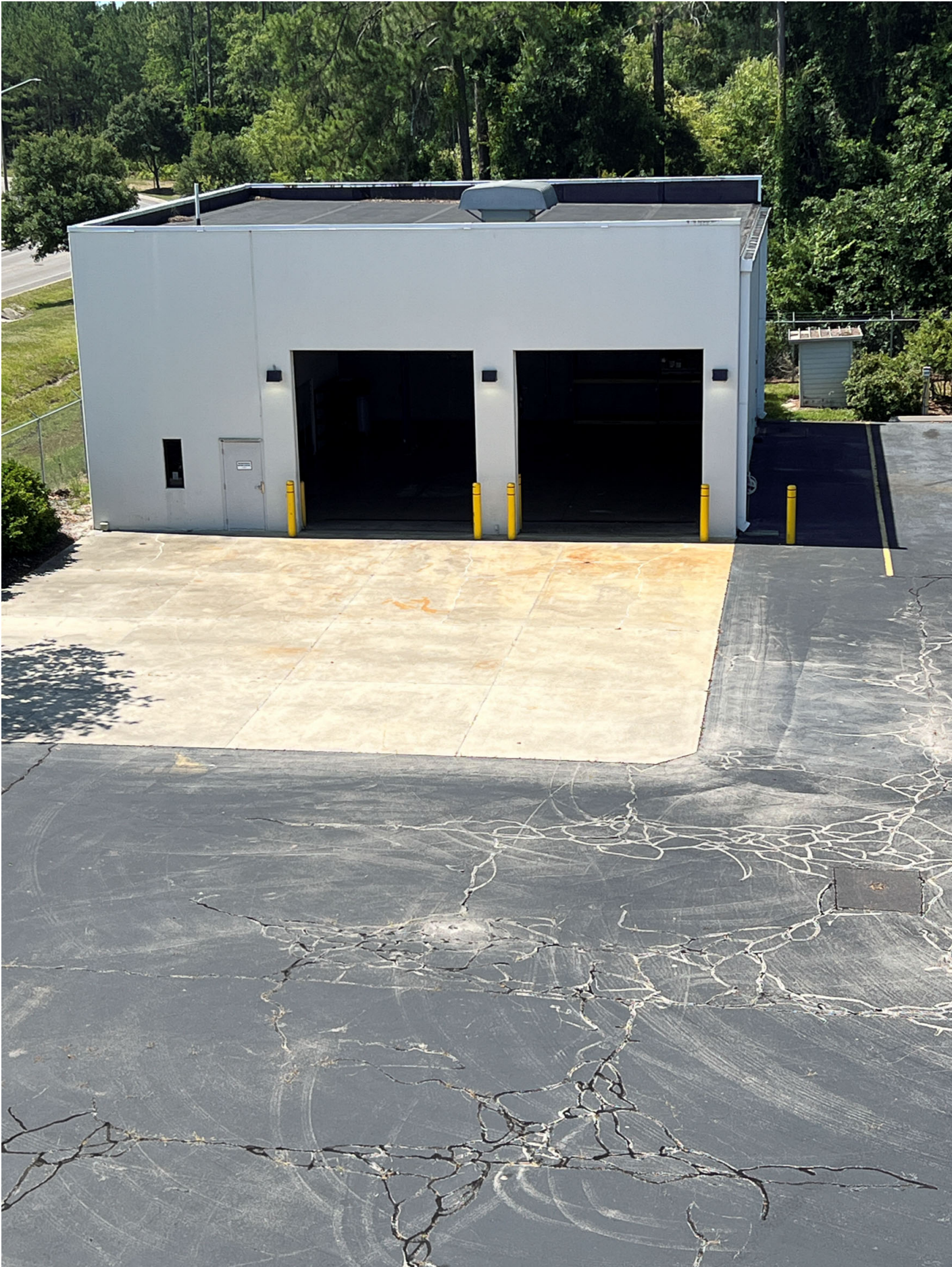
Freestanding maintenance / out building at southeast corner of site
