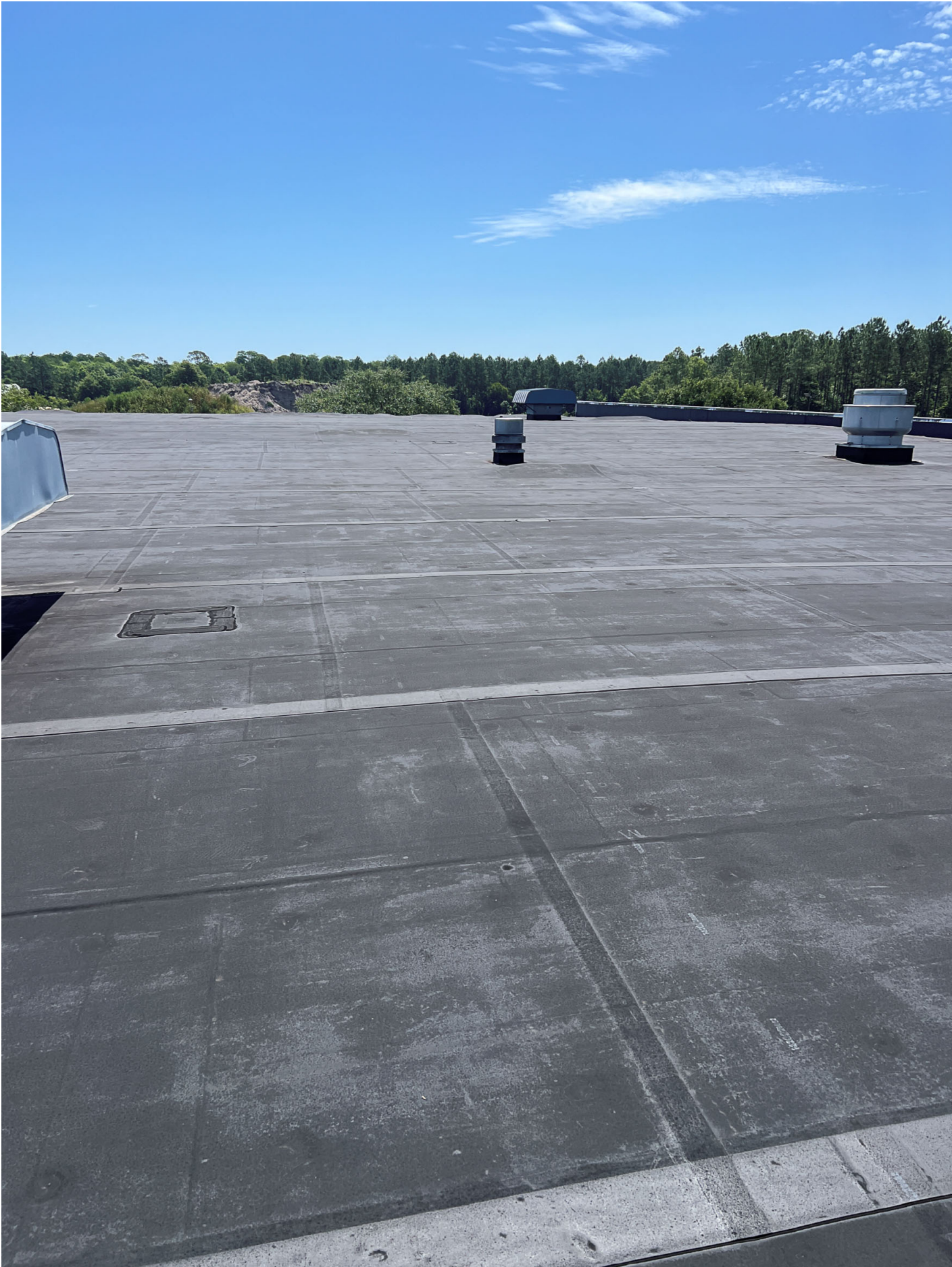
2000 warehouse roof viewing east/ roof exhaust fans / misc. paching / vapor bladders
