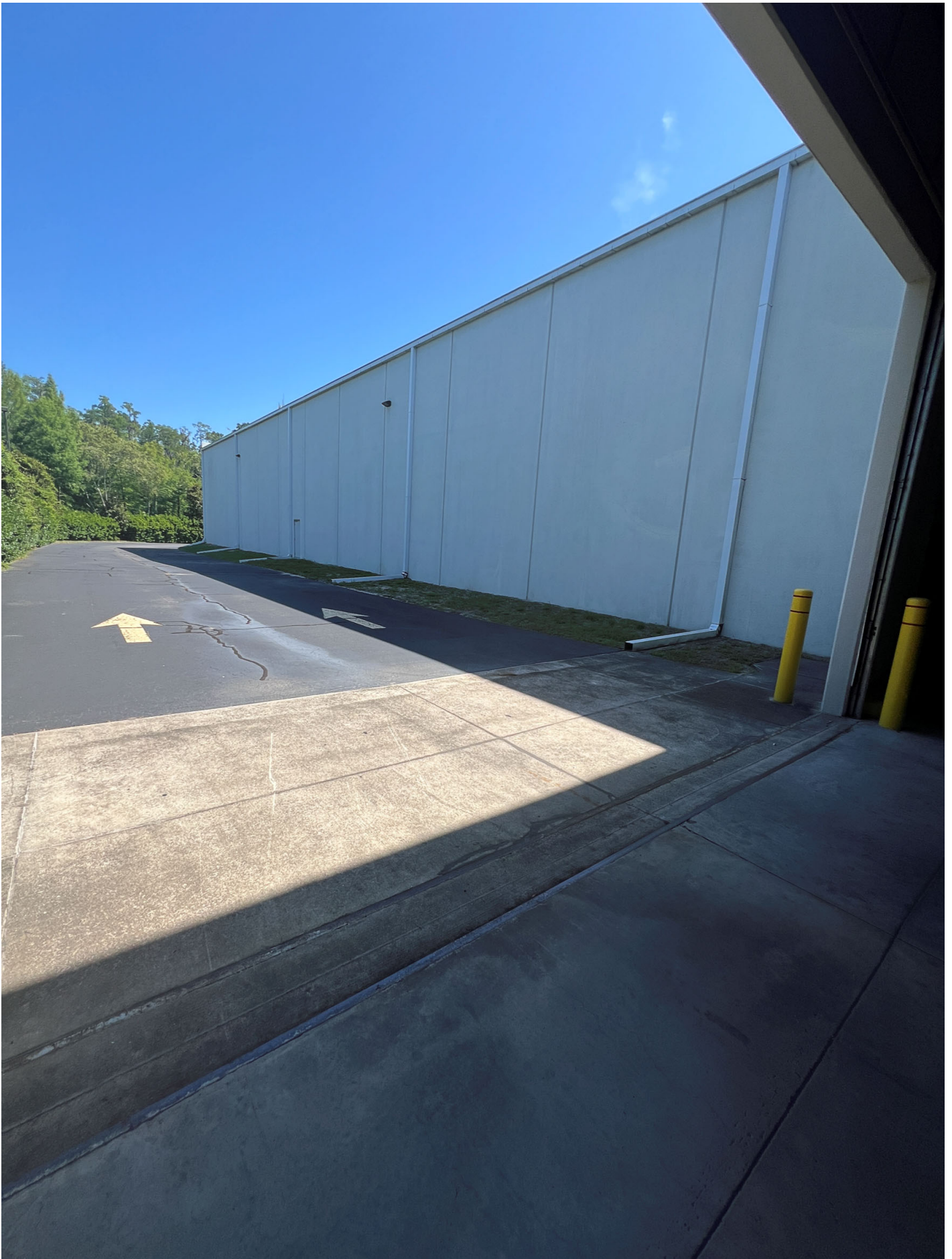
West side of the 2011 warehouse expansion
