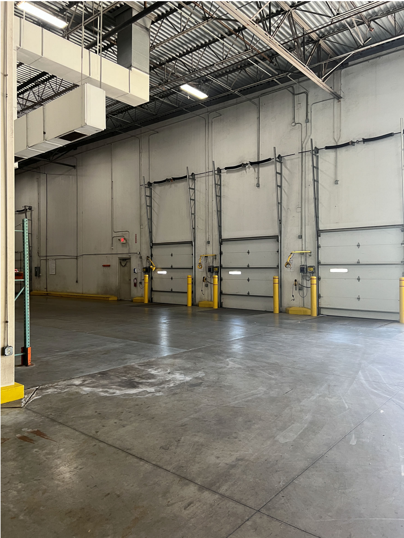
South recessed loading dock service doors
