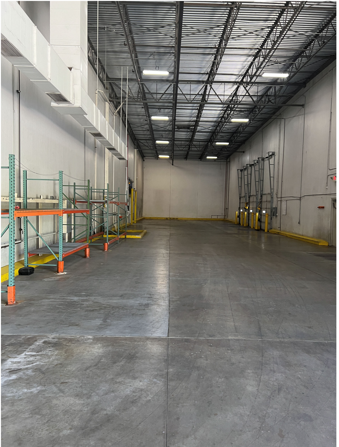
South storage / staging area for service truck loading at recessed loading dock
