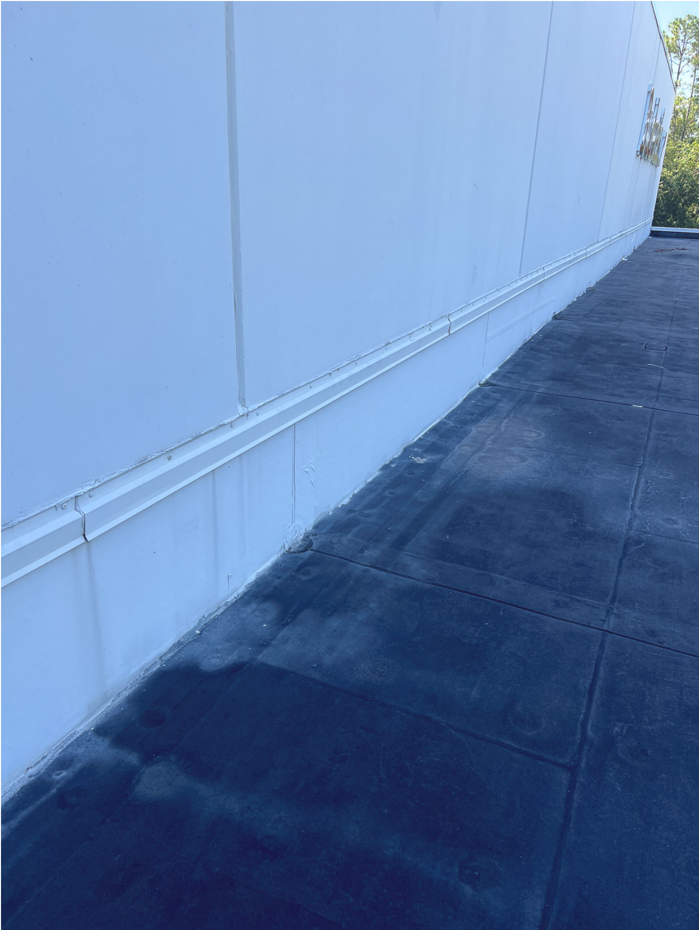
Lower to upper roof wall transition
