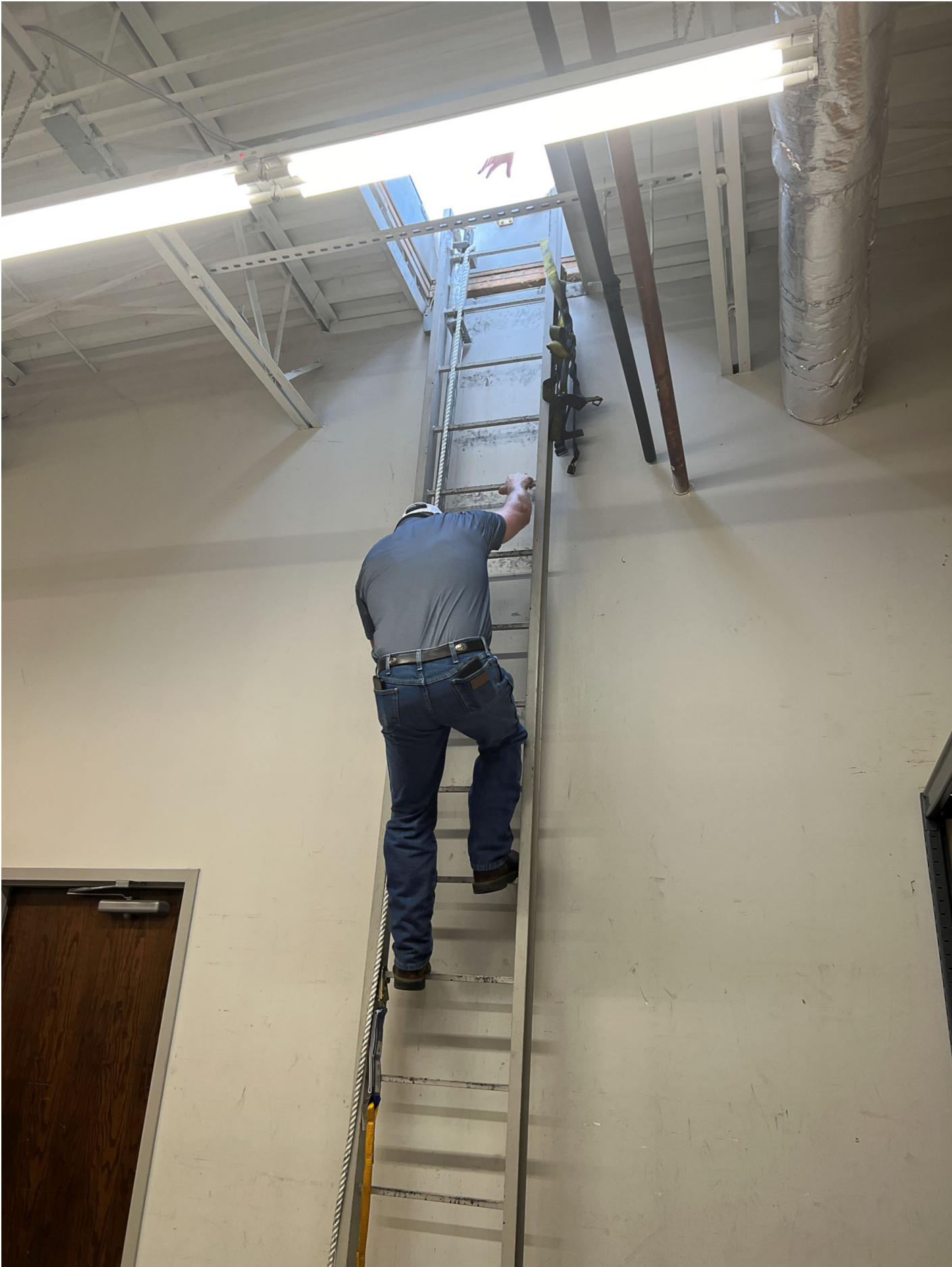
Access to the lower admin roof area
