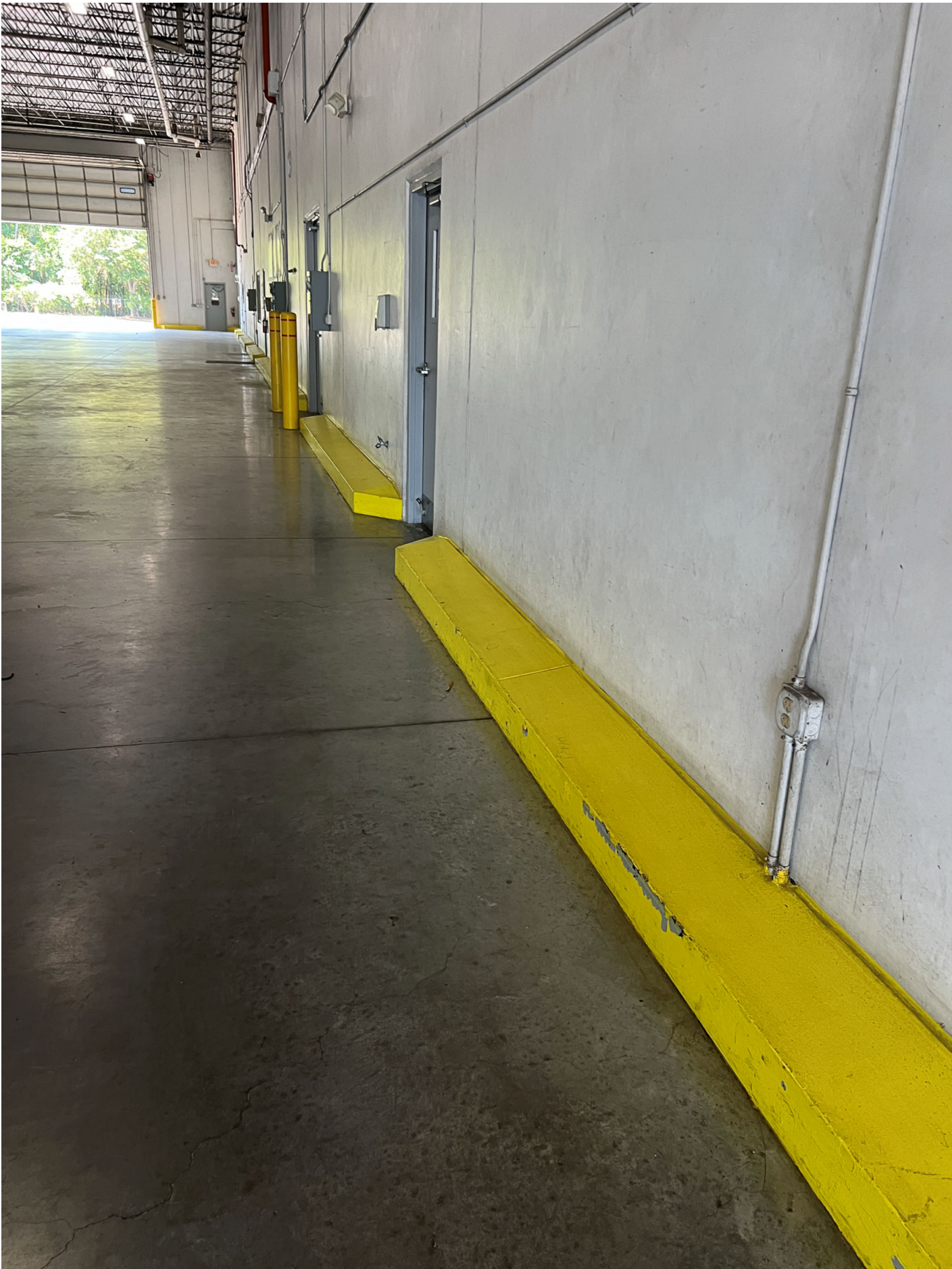
East wall of west drive-thru warehouse
