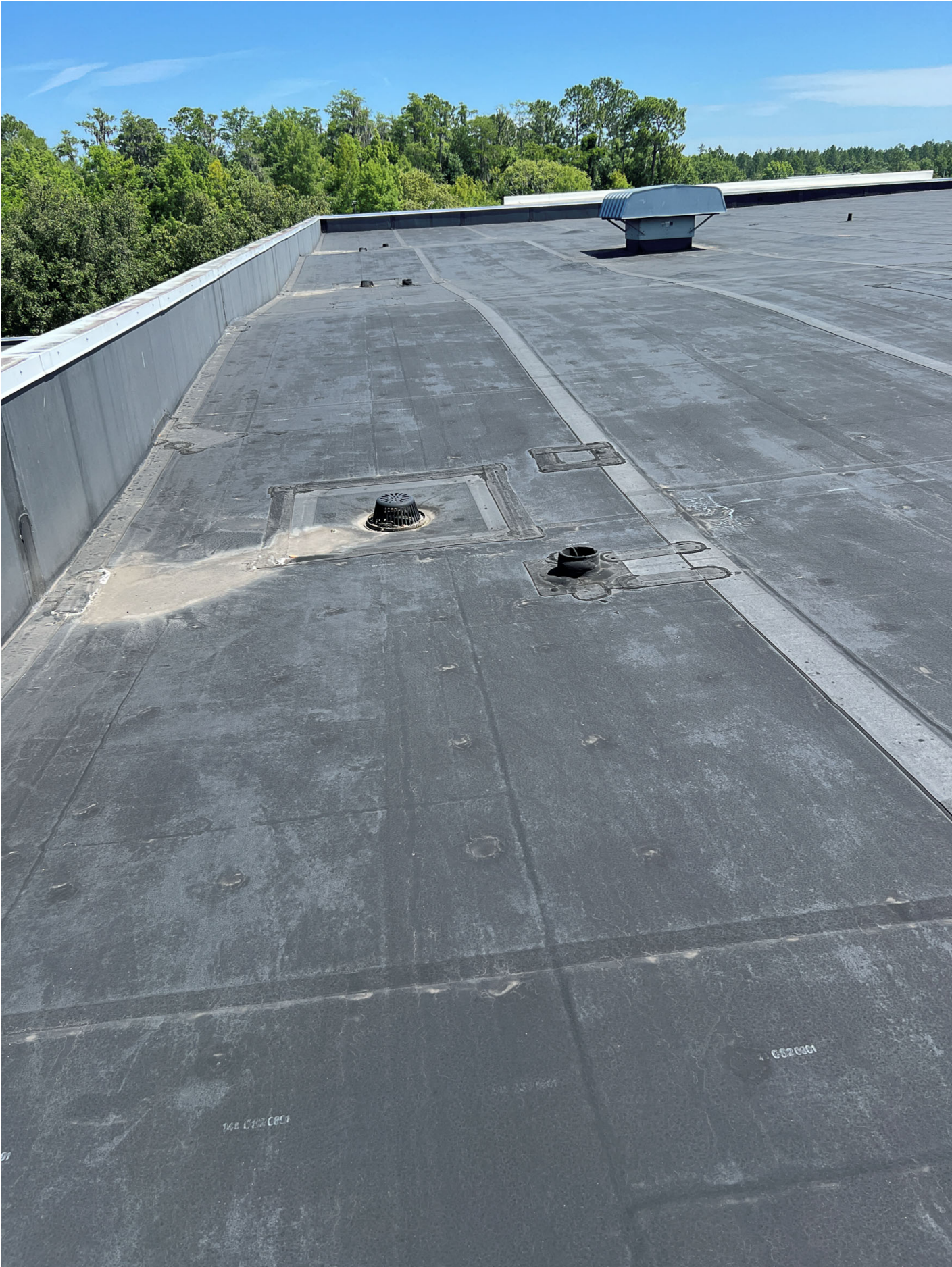
Upper 2000 warehouse roof east portion
