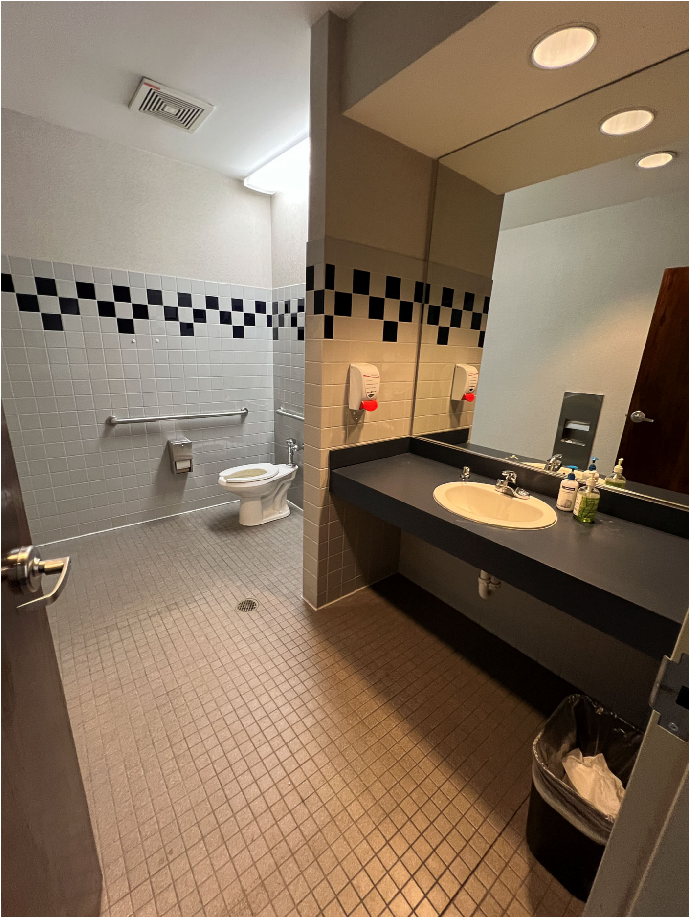
Male admin toilet room
