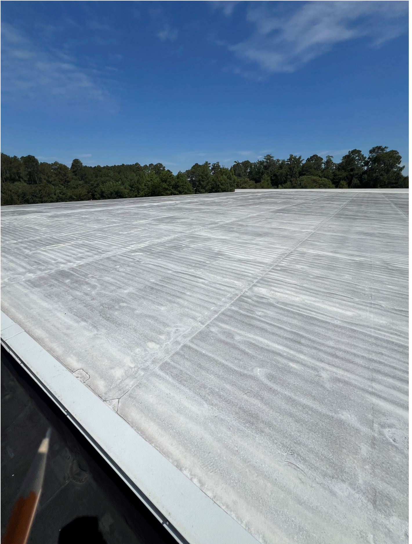
2011 warehouse addition with whole PTO single-ply roof membrane reasonable condition
