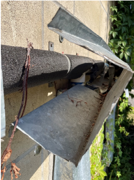
Figure 8: Shroud removed from the building
