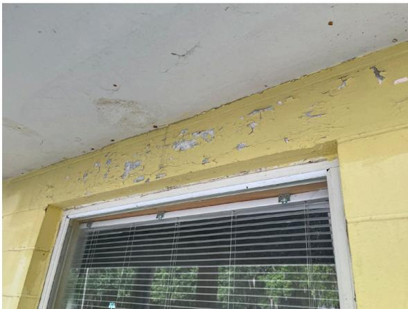
Figure 15 - Paint peeling on lintels above windows
