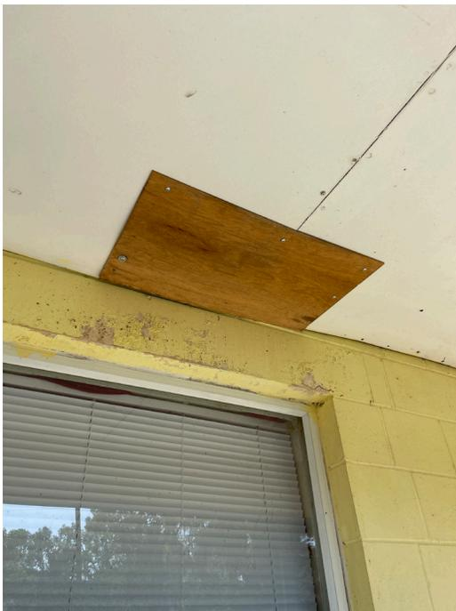
Figure 21 - Current condition of soffit in SW building
