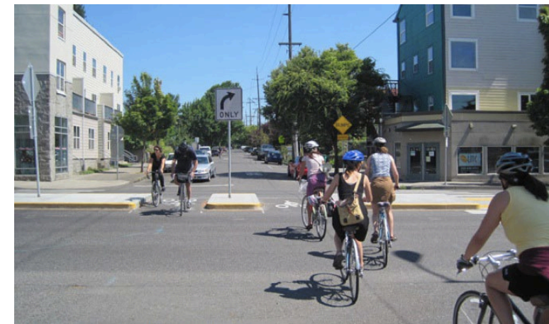
Median Refuge Island – Portland, OR A median refuge island and traffic diverter for a neighborway.
