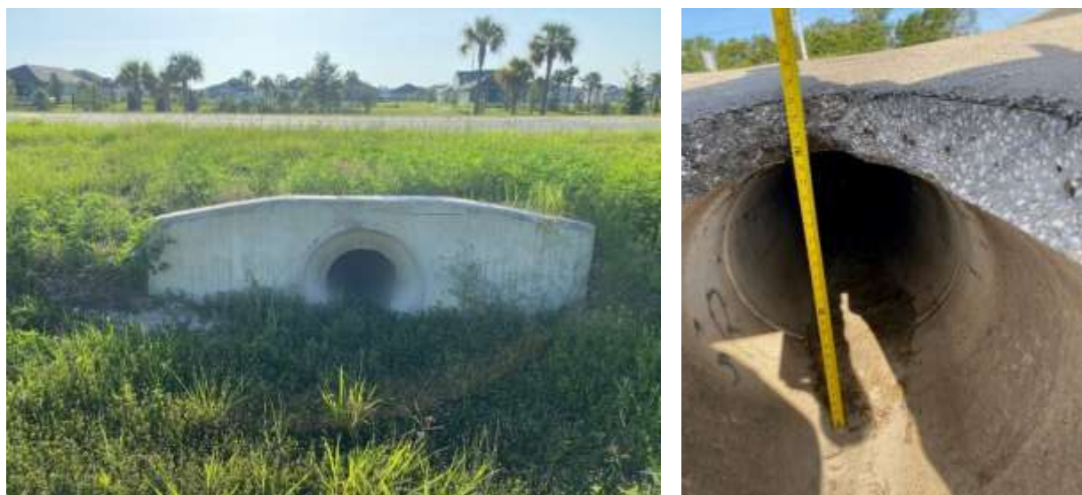
Figure 3 Stormwater Culvert Under Parker Road
