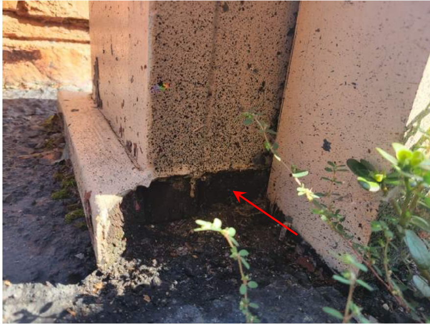
Photo 3: Rotting at wood column wraps
