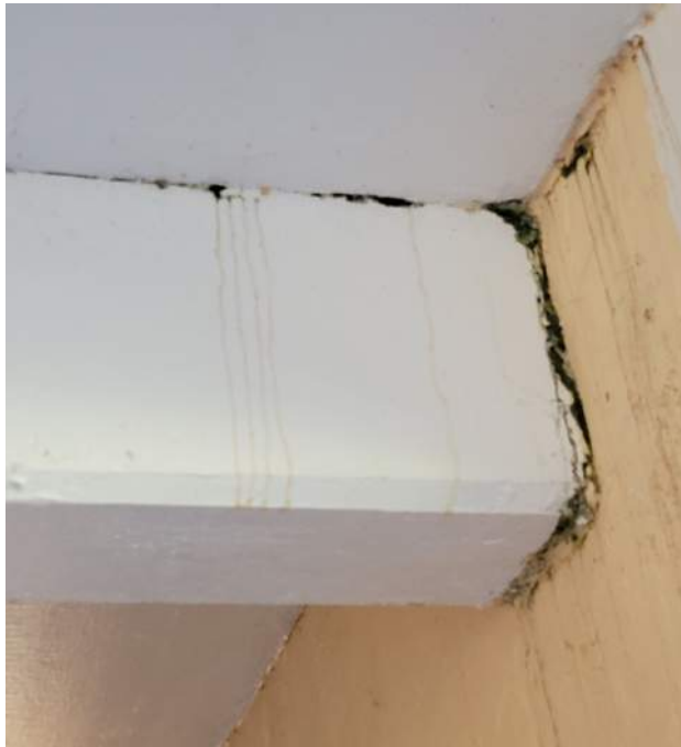
Photo 40: Moisture/Organic Growth at Exterior 2 nd Floor Beams
