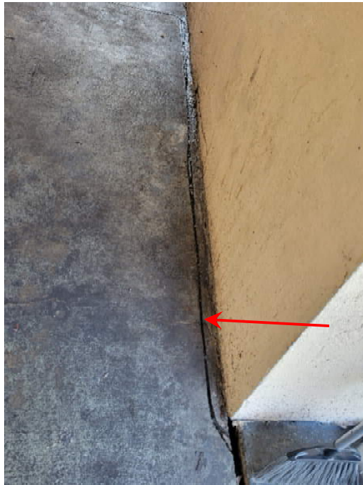
Photo 31: Concrete Cracking at 2 nd Floor Walkway
