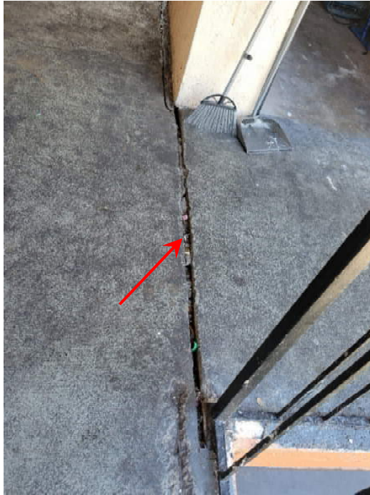
Photo 33: Unsealed Concrete Control Joint
