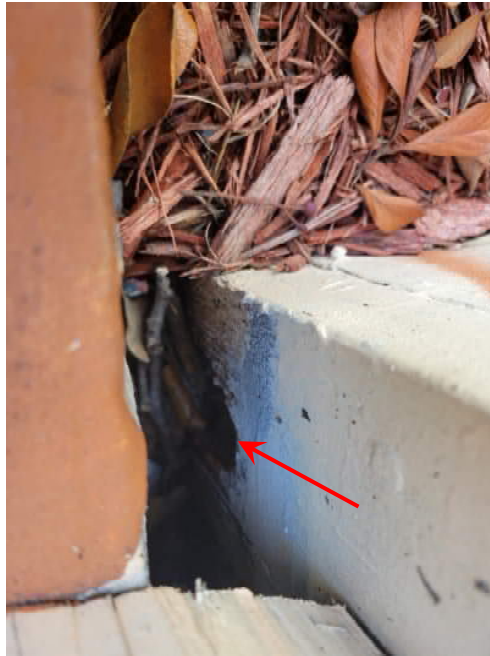
Photo 1: Rotting at drive-thru column bases
