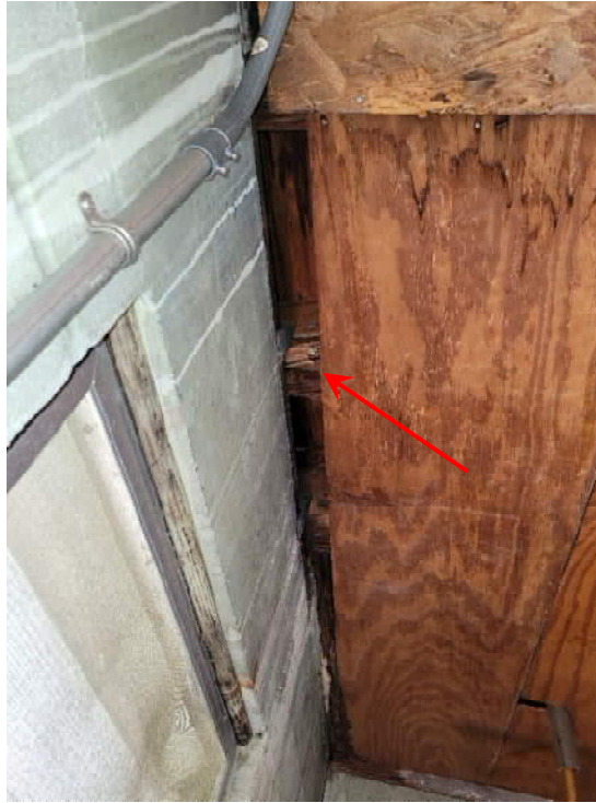
Photo 5: Rotting observed at exterior truss bearing and sheathing (mechanical room)
