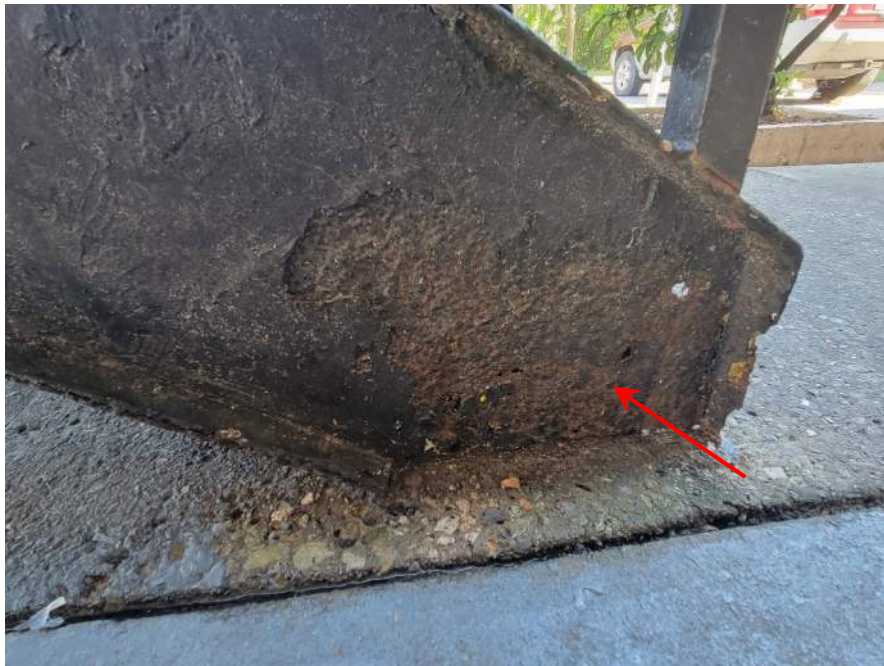
Photo 36: Corrosion of Exterior Steel Framing - Stair Stringer
