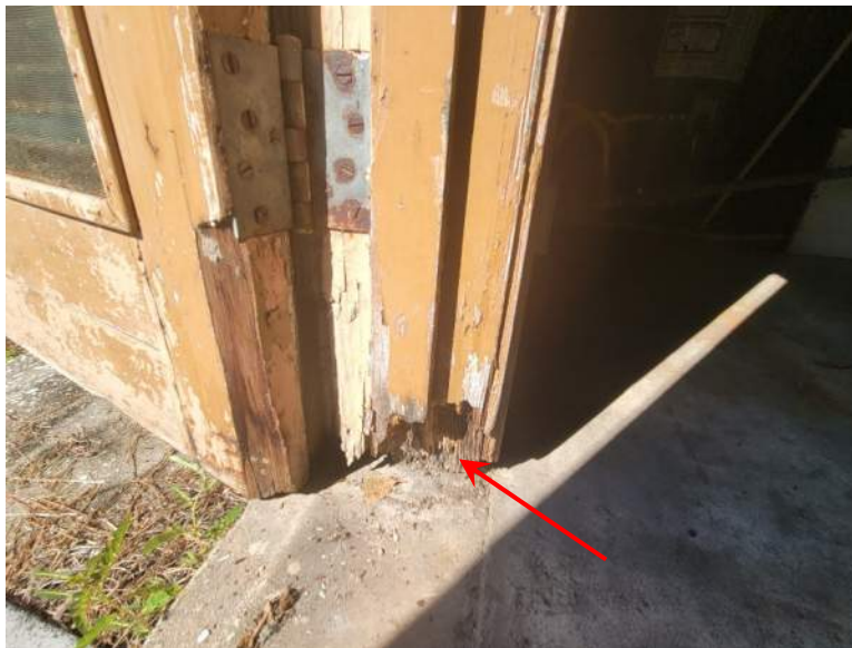
Photo 6: Rotting at Door Frame
