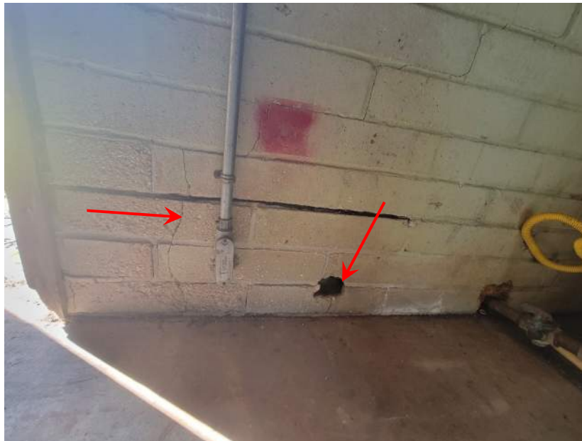
Photo 13: CMU Damage / Spalling
