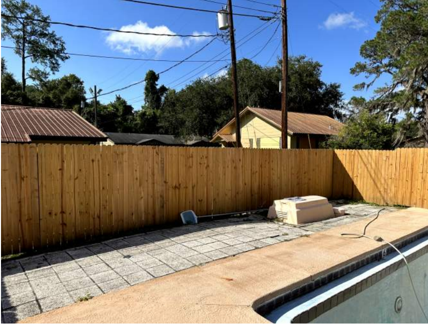
Condition: Irregular paver settlement adjacent to pool deck. Recommendation: Stabilize and compact grading below pavers and reinstall.
