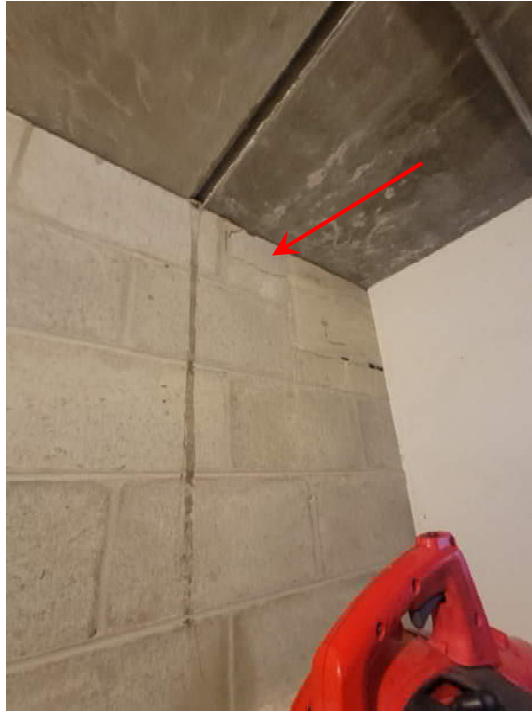
Photo 27: Damaged CMU Wall below Precast Concrete Planks
