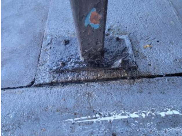
Photo 39: Missing/Corroded Anchor Rods at Exterior Steel Stair Post Base
