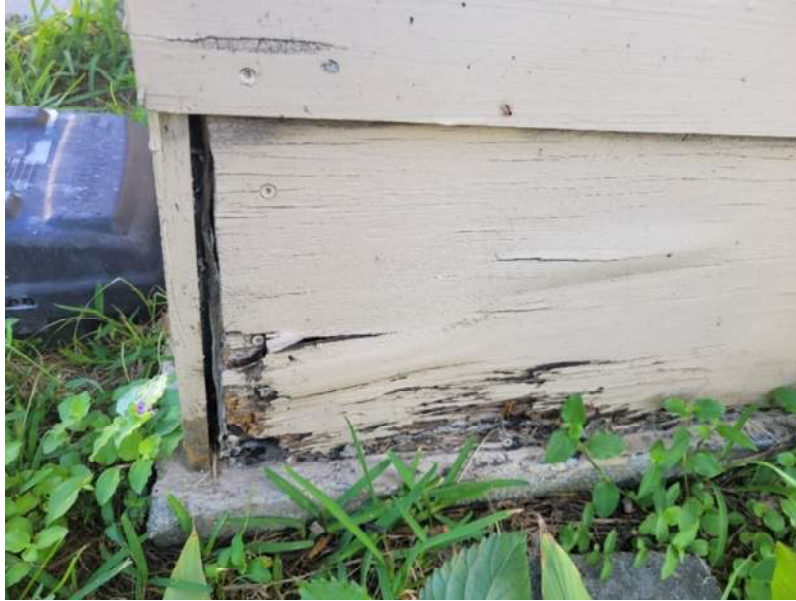
Photo 19: Rotting at Exterior Sheathing
