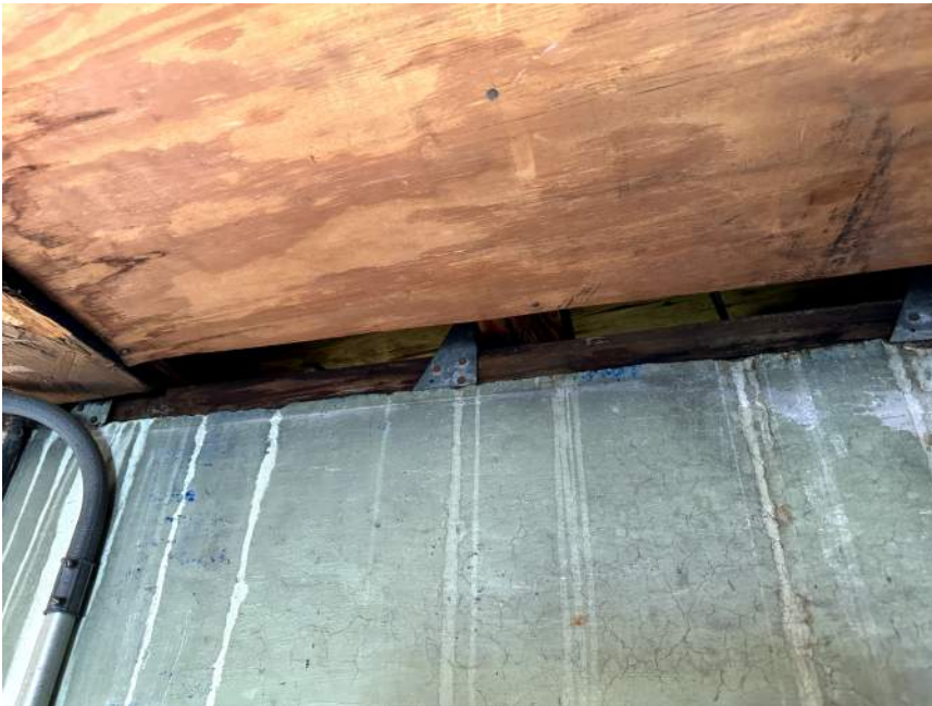
Condition: Evidence of moisture damage to truss sill plate. Plywood used for ceiling board has been damaged by water. Recommendation: Inspect all attic spaces for water damage and repair active leaks.
