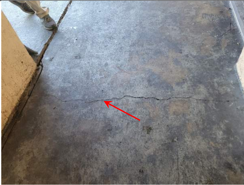
Photo 31: Concrete Cracking at 2 nd Floor Walkway
