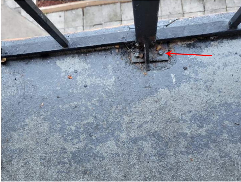
Photo 35: Corrosion at Guardrail Post Base Plate Anchors
