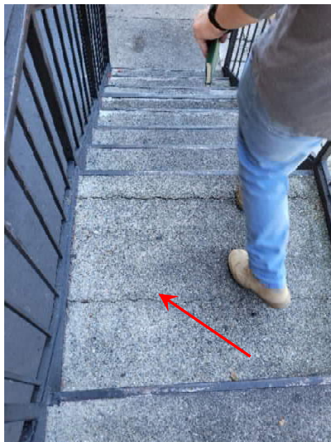
Photo 38: Cracked Concrete at Stair Landing
