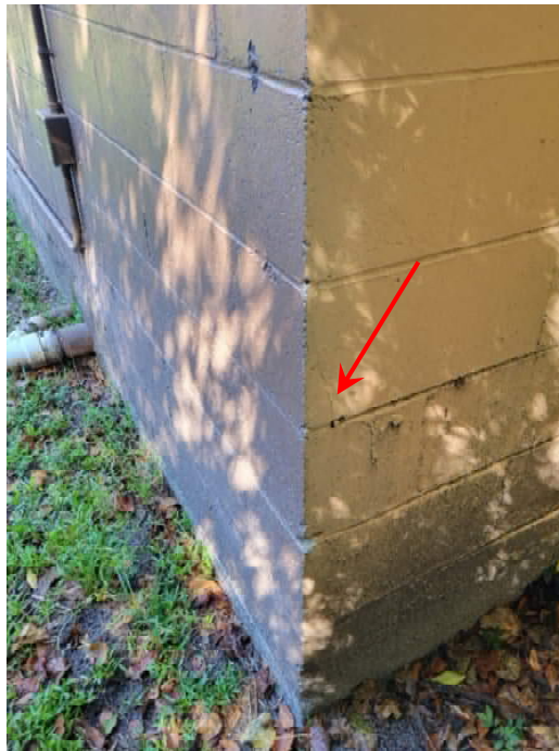
Photo 28: Cracking at Exterior CMU Wall
