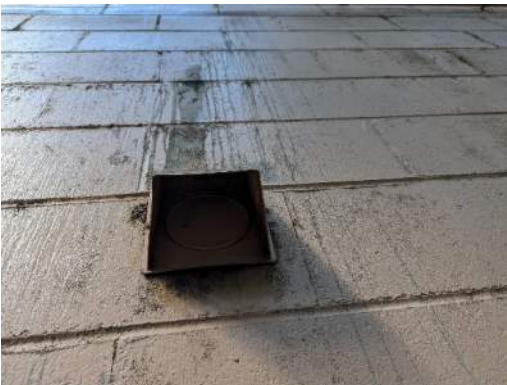
Two-Story Building Exhaust Wall Cap
