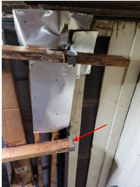
Photo 22: 2x4 Joists Supported by Straps in Tension
