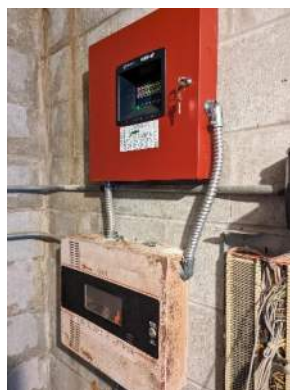
Two-Story Fire Alarm Control Panel
