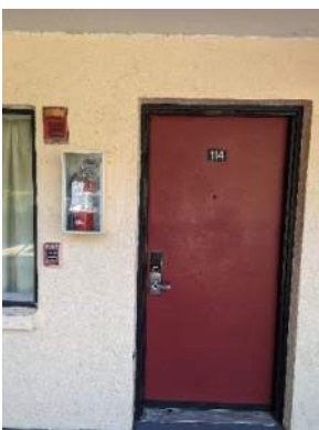
Two-Story Fire Alarm and Pull Station
