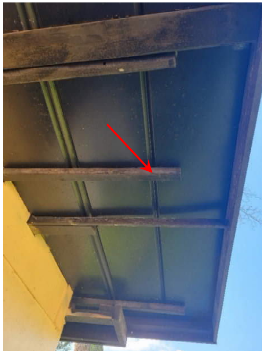
Photo 20: Cantilevered Purlins at Overhang
