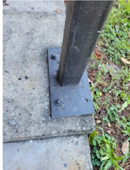
Photo 39: Missing/Corroded Anchor Rods at Exterior Steel Stair Post Base
