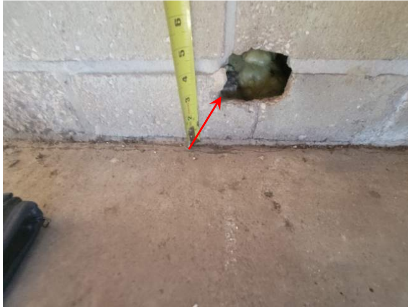
Photo 15: Unsealed holes in mechanical room wall
