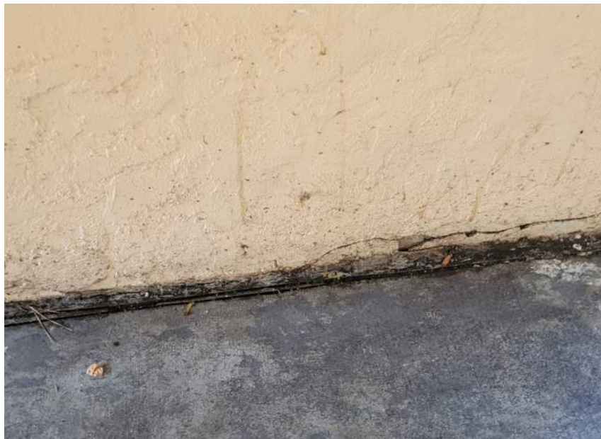
Photo 34: Failed Joint Sealant
