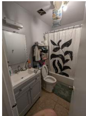
Apartment Bathroom with Inoperable Exhaust Fan
