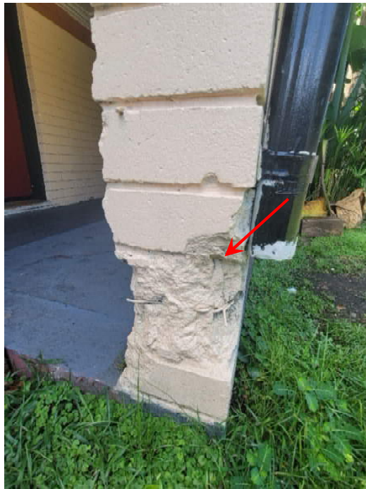
Photo 16: Damage to pilaster column at walkway
