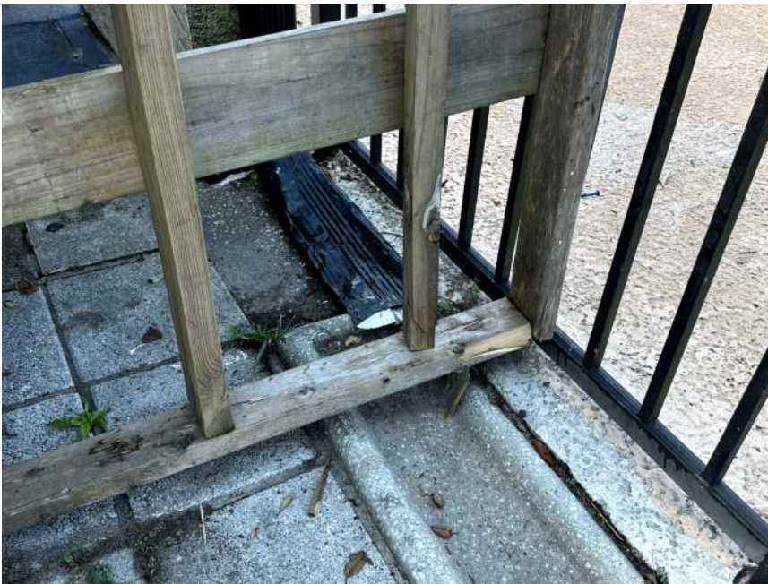
Condition: Downspout extension has been flattened. Recommendation: Replace extension.
