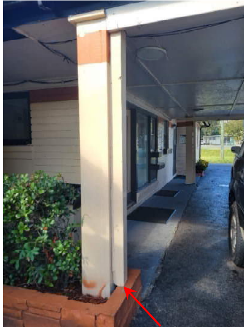
Photo 11: Wood repair post does not go down to the ground
