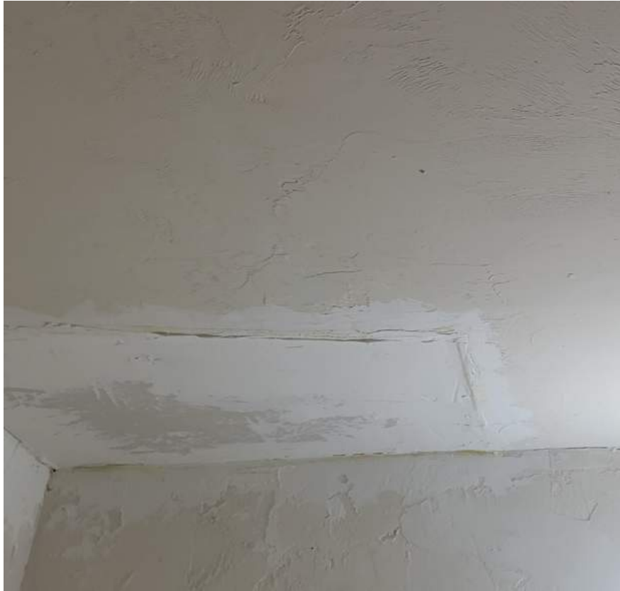
Photo 41: Sagging Plaster Ceiling at Roof
