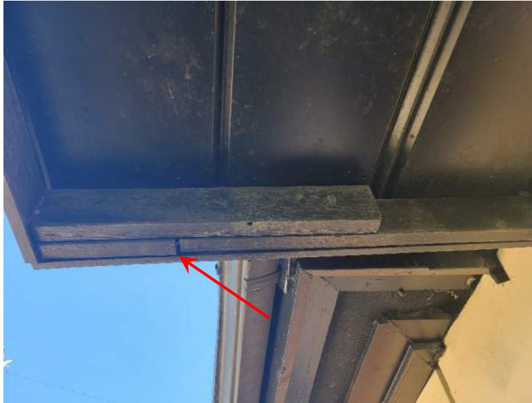
Photo 21: Splicing of Wood Outriggers
