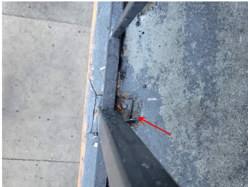
Photo 30: Concrete Spalling at Handrail Post Base
