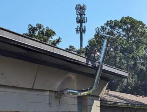
Office Water Heater Flue
