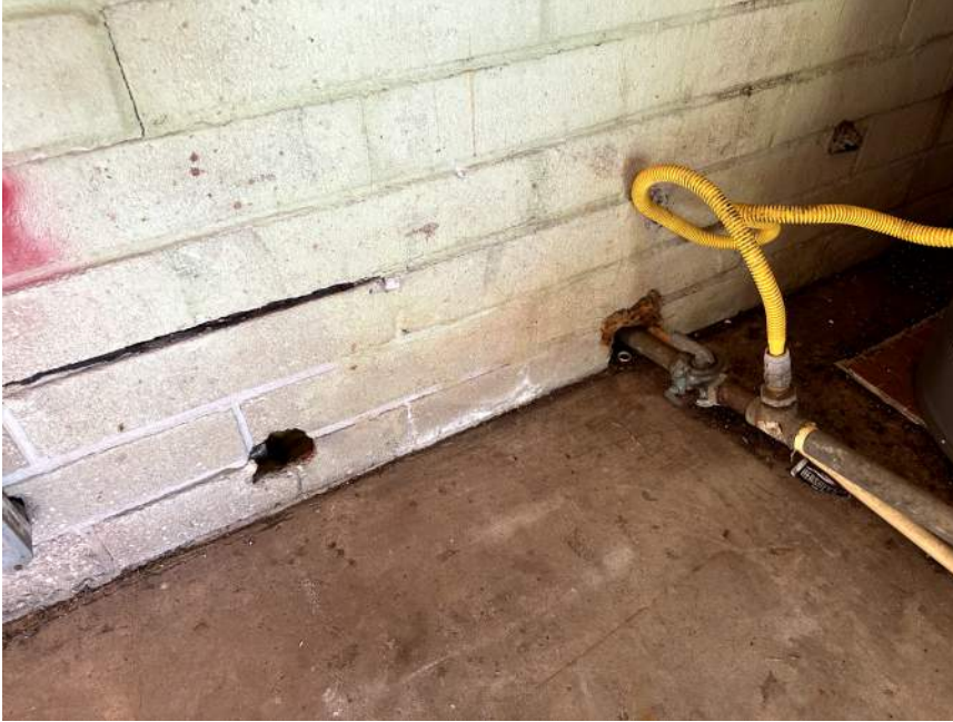
Condition: Hole in exterior wall CMU. Recommendation: Grout hole solid.
