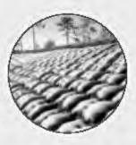
All Fabriform\* fabrics are manufactured with 100% continuous multifilament, high-tenacity nylon for stability and resistance to the strong alkalis present in concrete and are woven such that at least 50% by weight consists of textured fibers for optimum filtering characteristics and adhesion to mortar.
