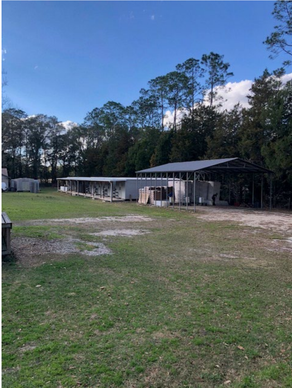
Photograph of unpermitted structures along northern parcel boundary
