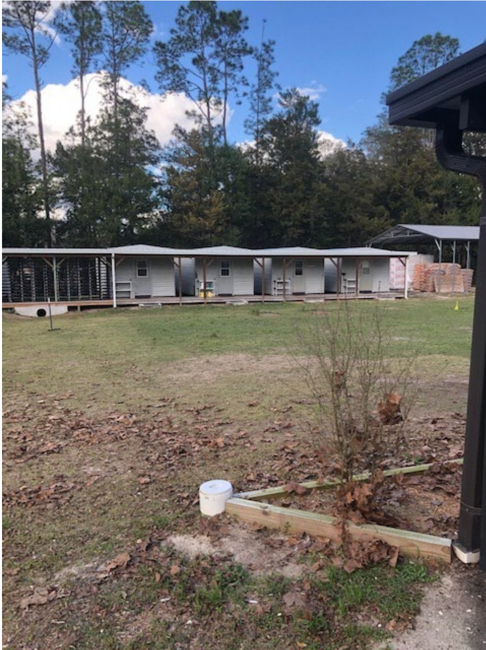
Unpermitted Accessory buildings containing breeding facilities
