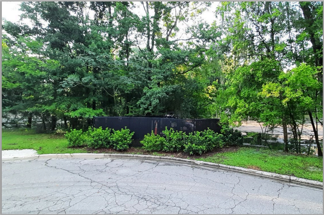
Single 8-inch pump with hard pipe, fencing and landscaping to reduce noise.
