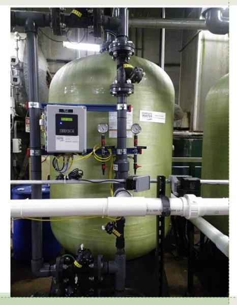
Typical Greensand Filtration Unit Source: Complete Water Solutions
