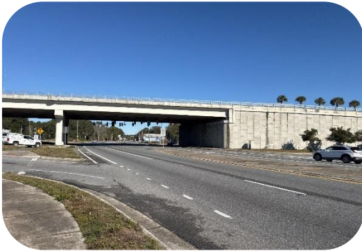
Interchange at US 301 &amp; Hawthorne Road
